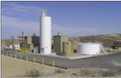
ASP stands for Alkaline Surfactant Polymer. An ASP Flood injects chemicals into a reservoir to "loosen up" stranded oil.
